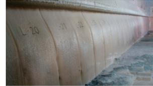
Fig.6 The photo of side wall blocks without unusual corrosion in Furnace-E.
