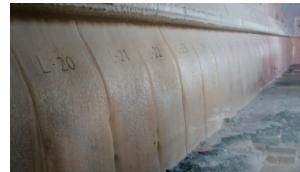
Fig.6 The photo of side wall blocks without unusual corrosion in Furnace-E.
